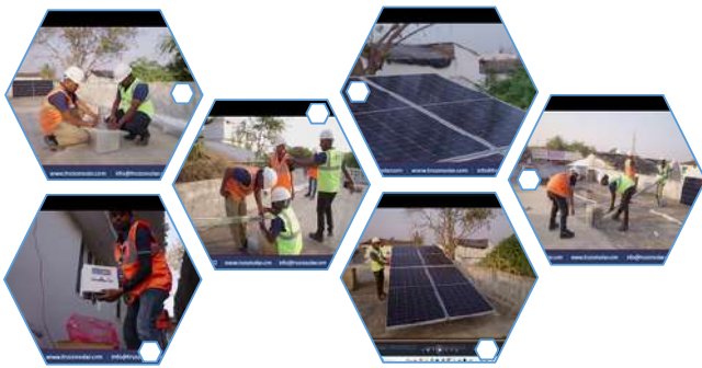
Truzon Solar has successfully installed Solar RTS at Kodang Constituency
